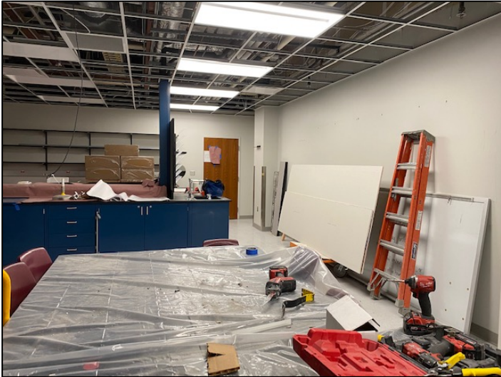
SL 144 under renovation.
